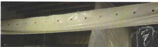
Plastic Bags are an Inexpensive Alternative to Metal Ductwork
